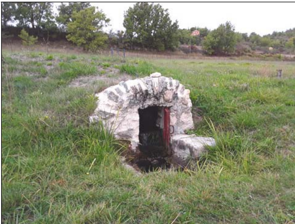
Station de surverse de la source.
